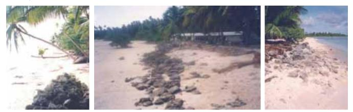
Figure 187 Erosion at end of seawall-Eita, Tabiteuea North. Figure 188 Collapsed seawall-Tewai school, Tabiteuea South. Figure 189 Collapsed seawall at Temotu island, Nonuti. (Source: Fig. 187 -189: Gillie, 1993).
