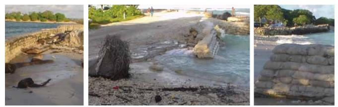
Figure 198 Erosion begins where wall ends. Figure 199 Erosion at end of seawall. Figure 200 Erosion seen at toe of sandbag wall.
