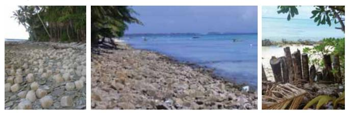
Figure 202 Collapsed Concrete cube Seawall at Nanumaga. Figure 203 Collapsed Concrete cube revetment at Funafuti. Figure 204 Collapsed Gabion basket wall and Tree Trunk wall at Nukulaelae. (Source: Fig.203: Tuvalu NBSAP)
