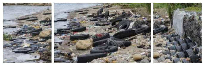
Figure 182 Tire wall collapsed at end of seawall. Figure 183 Tire wall was ineffective. Figure 184 Vehicle tire wall at end collapsed
