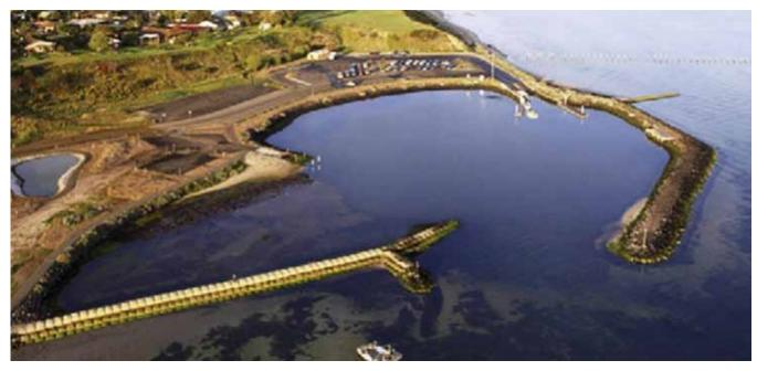
*Figure 24: Geotextile Sand-filled Container (Elcorock) Breakwater Example Source: (Hornsey, et al., 2011)*
