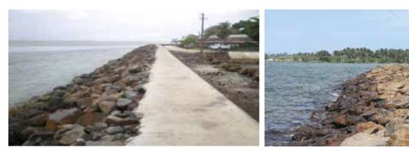
Figure 137 Partial concrete revetment at Piula. (Source: Fig.137 - 138: Moira Faletutulu)
