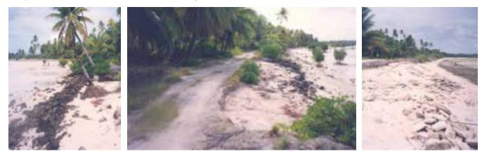
Figure 190 Collapsed wall at Rotima, Nonouti. Figure 191 Eroded road and seawall collapsed at Rotima..Figure 192 Collapsed concrete filled sandbag wall at Nonouti. (Source: Fig.190 - 192: Gillie, 1993).
