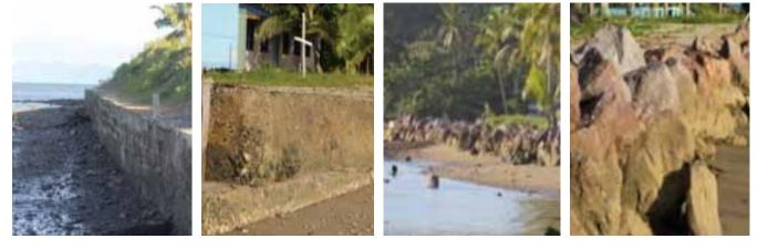
Figure 39 Navulivatu concrete seawall. Figure 40 Lomeri concrete wall. Figure 41 Lomeri Rock wall.
