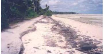
Figure 193 Collapsed seawall in Abemama. (Source: Fig.193-194: Gillie, 1993).
