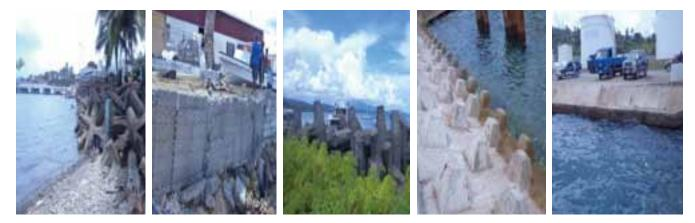
Figure 144 Breakwater structure. Figure 145 Gabion structure. Figure 146 Breakwater structure. Figure 147 Concrete revetment. Figure 148 Concrete seawall.
