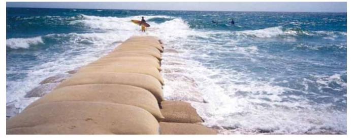
Figure 21: Geotextile Sand-filled Container (Elcorock) Groyne Example Source: http://www.elcorock.com/case-studies/maroochydore-protected-elcorock [Accessed 29 January, 2015]
