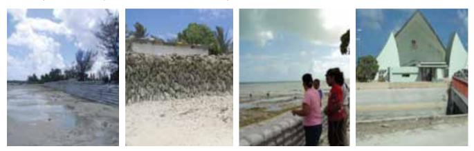
Figure 65 Concrete Sandbag wall. Figure 66 Rock wall. Figure 67 Causeway Concrete wall. Figure 68 Concrete revetment wall at Parliament House.
