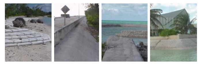
Figure 73 Mangroves and sand bags wall at Bonriki. Figure 74 Dainippon Causeway Bairiki to Betio. Figure 75 Private land-reclaiming project using sand bags wall at Bairiki. Figure 76 Sloping cement wall protecting Parliament House.
