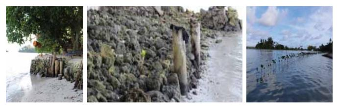
Figure 141 Rock Boulders seawall
