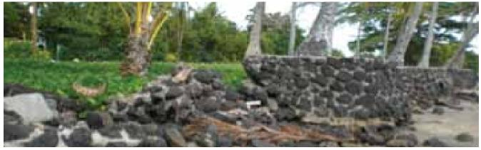
Figure 201 Collapsed seawall in Samoa (Source: Yamamoto and Esteban, 2011)
