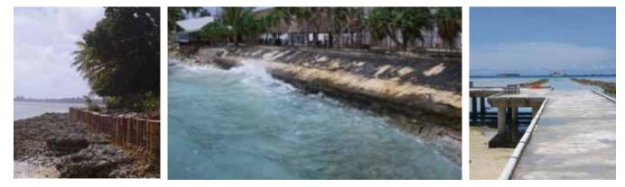
Figure 158 Private wall made up of 44-gallon drums filled with concrete. Figure 159 Concrete wall in front of Hotel. Figure 160 Nukufetau jetty and reef channel. (Source: Fig 158: Ms. Makereta Komai. Fig 160: Temata Shozo)
