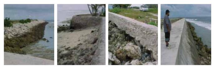
Figure 102 Rip rap rock revetment. Figure 103 Concrete wall. Figure 104 Long concrete wall. Figure 105 Concrete wall with rocks at basement. (Source: Fig.102 - 105: Maharaj, 2000).
