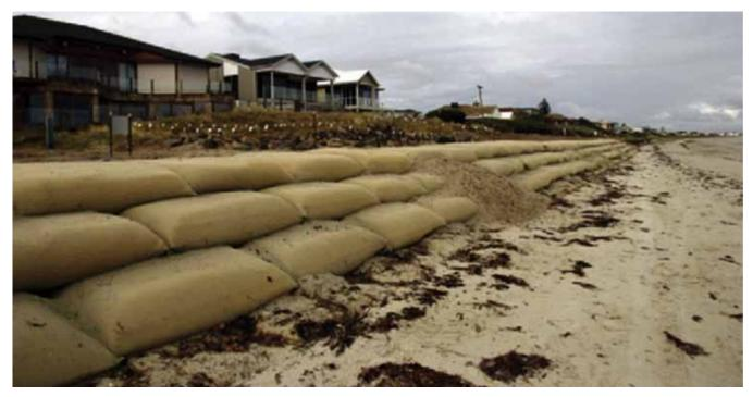
*Figure 23: Geotextile Sand-filled Container (Elcorock) Revetment Example Source: (Hornsey, et al., 2011)*
