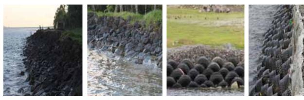
Figure 43 Naitonitoni rip rap rock wall. Figure 44 Naitonitoni rock wall. Figure 45 Lami rubber tire wall. Figure 46 Lami Gabion basket wall.
