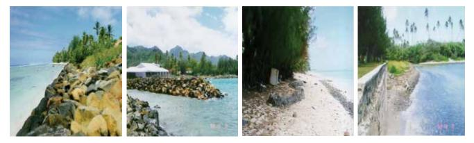
Figure 25 Rock riprap wall, Figure 26 Avarua rock groynes, Figure 27 Gabion basket wall, Figure 28 Ngatangiia concrete wall (Source: Fig.25-28: He, 1999).
