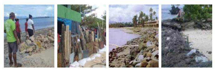
Figure 133 Stone wall at Mou Kele village. Figure 134 Sandbag and tree trunk wall. Figure 135 Rock wall at Gilibwa village. Figure 136 Gabion Basket wall at Los Negros Island.
