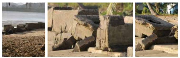
Figure 179 Part of seawall at Lomeri High School collapsed. Figure 180 Same seawall looking from seaside. Figure 181 Poor engineering work
