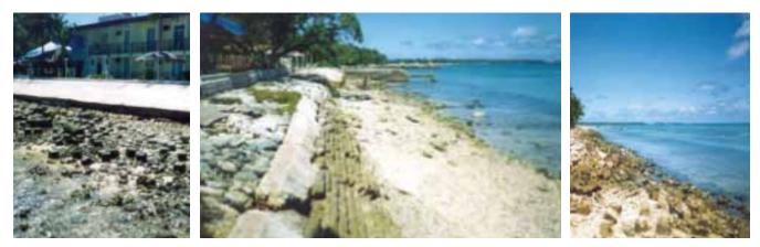
Figure 205 Damaged boulders at toe of concrete seawall, Funafuti. Figure 206 Damaged seawall at Vaiaku Lagi Hotel. Figure 207 Collapsed concrete cubes revetment. (Source: Fig. 205 - 207: Xue and Malologa, 1995).
