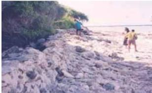
Figure 194 Collapsed seawall in Kuria.
