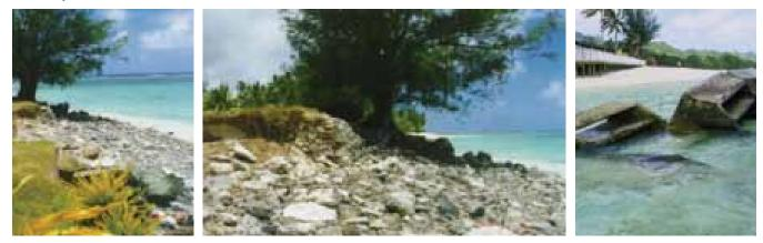
Figure 176 Sea erosion caused by failed seawall. Figure 177 Collapsed seawall in Cook Islands. Figure 178 Collapsed groyne at west end. (Source: Fig. 176 - 178: He, 1999)
