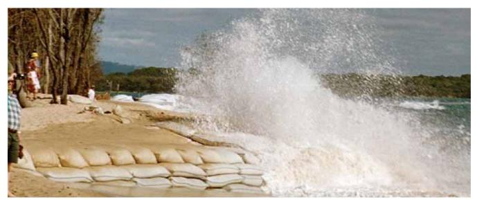
Figure 22: Geotextile Sand-filled Container (Elcorock) Seawall Example Source: http://www.elcorock.com/case-studies/maroochydore-protected-elcorock [Accessed 29 January, 2015]
