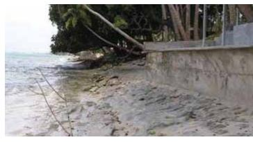
Figure 97 Seawall placed on rock. (Source: Fig.97 - 98: Murray Ford and Coastal Consultants NZ Ltd, 2013)
