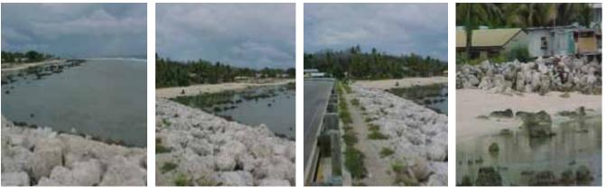
Figure 106 rock revetment.Figure 107 layout of rock revetment.Figure 108 rock wall.Figure 109 ro(Source: Fig.106 - 109: Maharaj, 2000)
