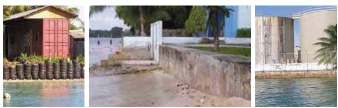
Figure 99 Vehicle tire neatly stacked as seawall.Figure 100 Concrete wall.Figure 101 Seawall protecting oil tanks.(Source: Fig.99 - 101: Murray Ford and Coastal Consultants NZ Ltd, 2013).Figure 101 Seawall protecting oil tanks.
