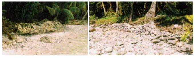
Figure 185 Polap Island erosion at toe of seawall. (Source: Fig 184 -185: Maharaj, 1998).
