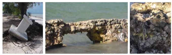
Figure 195 Erosion of important monument. Figure 196 Remains of stone wall. Figure 197 Gabion basket -broken wire.
